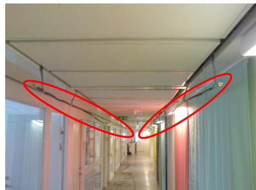
Photograph of two leaky feeders installed beneath the suspended ceiling in the corridor.
